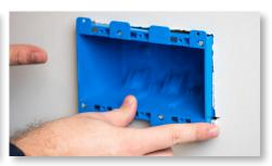
Designed specifically for cutting out 3 and 4-gang non-metallic old work boxes, this wall template level is perfect for ensuring the boxes are level every time. This wall template level features the following:
