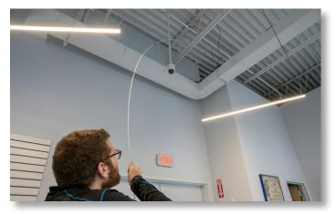
Designed to facilitate telecom and datacom installations, this glow rod is the perfect tool for pushing and pulling cables in low light applications. These glow rods feature the following:
