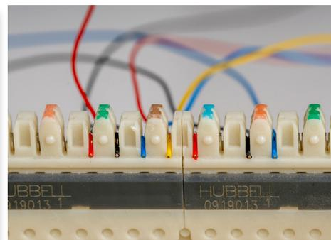
Designed to terminate 4 pairs of wires simultaneously, this punchdown tool is perfect for terminating multiple wires on 110-terminal blocks quickly and easily. This punchdown tool features the following:
