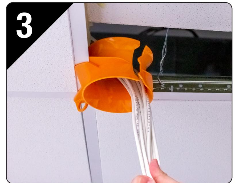
3. With the ceiling grid slotted between the Cable Funnel's tabs, push until the Cable Funnel locks into the corner. You are now ready to run your wires!
